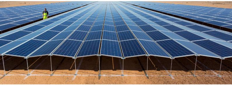
The patented PEG<sup>®</sup> substructure has only rods and plates, without rails and crossbeams, with the module frames practically part of the substructure.
