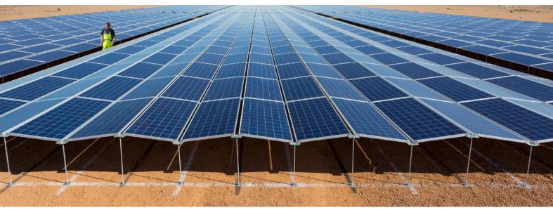
The patented PEG® substructure has only rods and plates, without rails and crossbeams, with the module frames practically part of the substructure.
